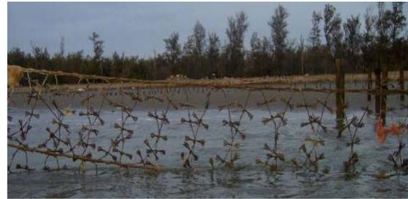
Fig. 8. Short wire fins attached to the wire nets of No. 2 flexible breakwater.
