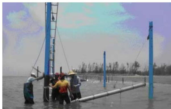
Fig. 6. Assembling the concrete posts with spring-pipes.
